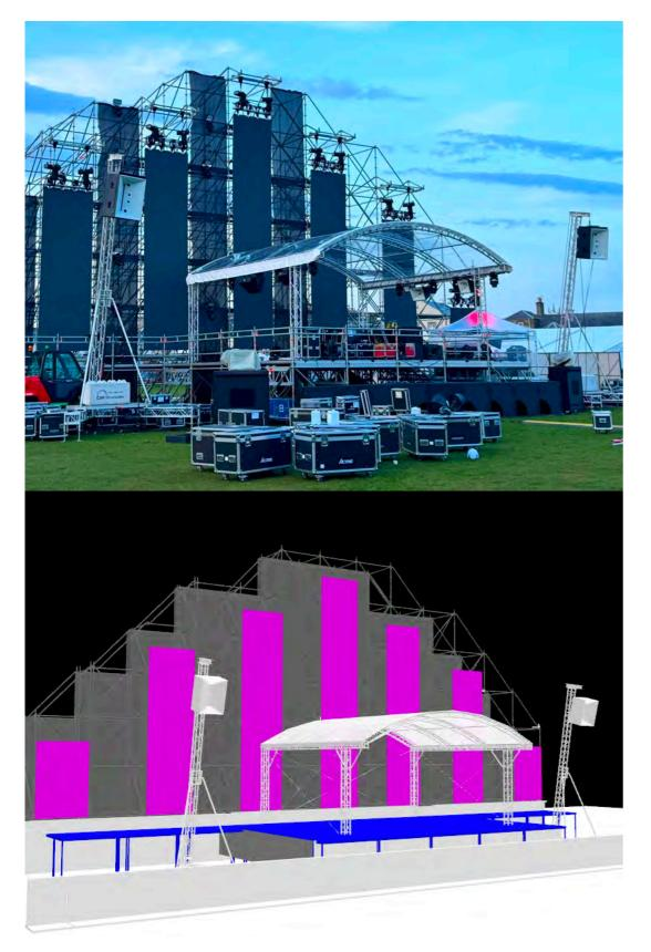
With an efficient setup time, modular design and versatile rigging options, our 8x6 stage can be customised to suit your event's specific needs. It comes standard on a 750cm or 4ft leg system. To add height to the structure, video towers, or when dealing with challenging site conditions, our structures can be constructed on a fully modular Layher substructure.
